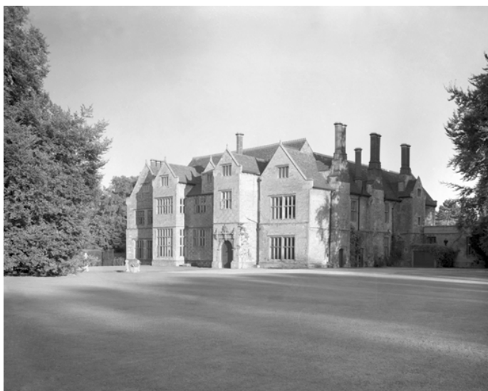
Fig 5 Sawston Hall, Grade 1 Listed Tudor Manor house
