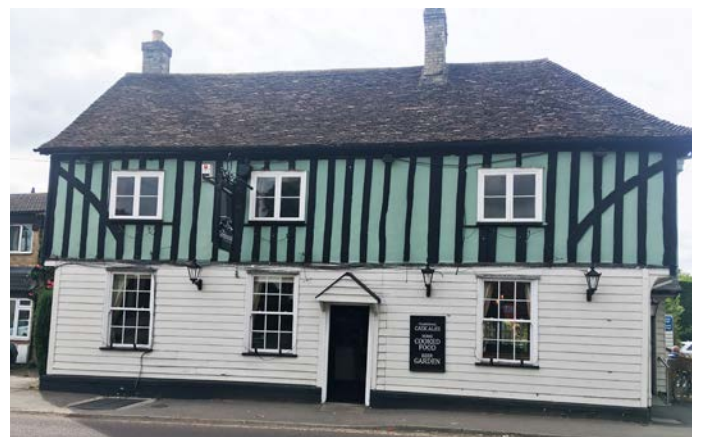
Fig 51 High Street frontages - Renovated pub
