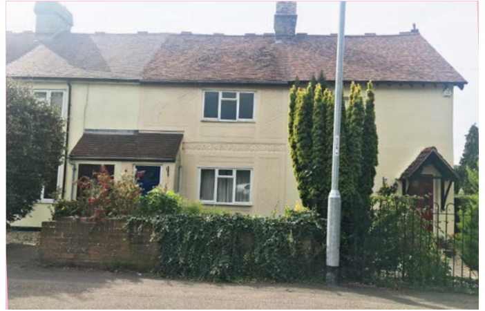
Fig 12 Terraced homes with lime render detail
